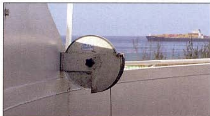
The Retractable Grounding Assembly reduces the risk of fires sparked by lightning. (Image courtesy of Lightning Eliminators)
